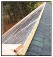
Adding Insulation To An Existing Roof: RAYCORE's lightweight, easy to use, modular roof panels with integrated framing member or "studs" is the perfect solution for adding insulation to the roof of an existing structure without disturbing the interior of the home. Simply frame the edge of the roof extending fascia and soffits and apply panels to existing roof. Deck as required, and apply roofing in an appropriate manner.
