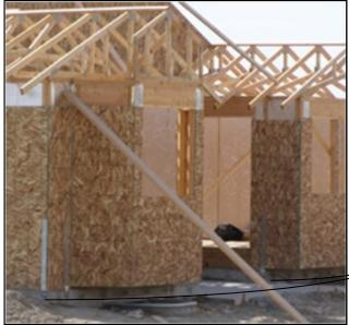
Hurricane Straps example (ie. Simpson STHD straps). As you would with conventional stick framing, hurricane straps are nailed into the RAYCORE Wall Panel's integrated studs. If the integrated stud in the panel does not line up with the STHD strap then you will need to place a stud in proper location during the framing process.
