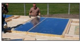
frame your first corner. Start laying panels out, cutting panels when necessary. When your wall meets a door or window simply cut the panel so it butts tight against the king stud on the window or door frame, and use cut material to continue on the side opposite the opening, cutting where
