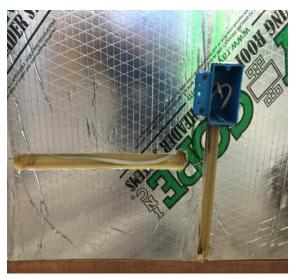
Place wires in the chase. Once inspections have been performed and rough wiring has been approved, backfill channels and penetrations with polyurethane canned foam. Once cured, remove any excess foam and cover with a vaporproof airsealing tape to ensure an airtight seal. This ensures the safety and efficiency of the electrical wiring system while maximizing the energy efficiency of the wall panel system.
