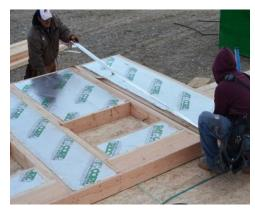
with vaporproof air-sealing tape. For best results, RAY-CORE recommends the using compatible FSK tape supplied by RAY-CORE. Take care to prevent damage to the panels and their foil facing during handling. However, if small tears, occasional bumps or gouges occur, they can be easily repaired by filling with canned polyurethane foam, flexible caulk, and/or by applying vaporproof air-sealing tape. This will ensure the long-term efficiency and reliability of the wall assembly.
