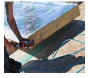
To ensure an air-tight joint, apply a continuous bead of foam-friendly construction adhesive or polyurethane canned foam to all edges, between the panels and all other framing members to seal joints. Push panels firmly together, ensuring there are no gaps and that the panels are tight and square. Attach the panels to the roof structure as instructed in Step 3. If further sealing is required, do so once the panels are permanently attached to ensure an air-tight structure.
