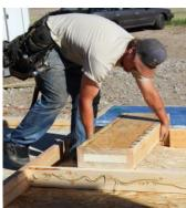
Step 2. Wall Layout: Begin by establishing your layout, starting with the corners (see Step 3 & 4). Place lumber, measure, and mark the top and bottom plates. Lay out panels, door and window frames, etc., according to your design plan. This step ensures accurate positioning and alignment of structural components before assembly.
