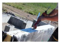
Step 5. And You're Off! Apply a continuous bead of construction adhesive or polyurethane canned foam to sides of the RAYCORE Wall Panel and adjoining framing members. This will adhere the panels and provide an airtight seal. Push the panels firmly together so that the foam side of one panel touches the wood side of the adjoining panel, maintaining your layout. Ensure that the panel joints are tight and square at all times to eliminate air infiltration, and prevent
