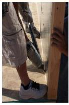
Construction process and project requirements. Apply a continuous bead of foam-friendly construction adhesive to the bottom plate to create an airtight seal between the subfloor and the wall. Securely face nail the bottom plate on both sides to the rim board and floor joists using appropriate fasteners per conventional framing practices and building code requirements.
