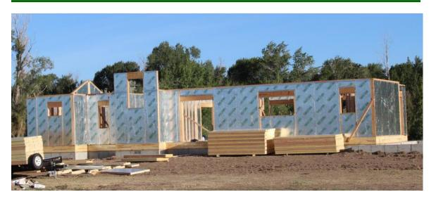
RAYCORE Structural Insulated Wall Panels® are not intended to serve as a finished and exposed surface. Internal surfaces of panels must be covered with a minimum 15-minute thermal barrier, such as 1/2 inch (12.7mm) gypsum wallboard or other approved materials. External surfaces of the panels should be finished promptly with materials that offer protection from sunlight, weather, moisture and all other elements. This ensures the longevity and performance of the wall system.
