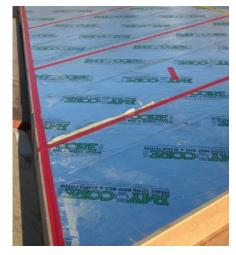
To achieve optimal performance and further prevent air infiltration and vapor transference, seal all seams, joints to additional framing members, and penetrations with vaporproof air-sealing tape. For best results, RAY-CORE recommends using compatible FSK tape supplied by RAY-CORE.
