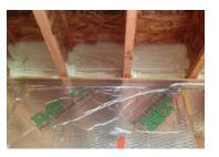
effectiveness. Although spray foam is not the best insulation choice, it is a very good air sealer. Consider adding 2 to 6 inches (50 to 152mm) of polyurethane closed cell spray foam, installed by an experienced installer, to each floor's rim board and back it with additional insulation whether it be fiberglass, cellulose, rockwool or even better, RAYCORE panel scraps to achieve at least an R-value equal to that of your walls.
