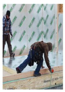
bead of construction adhesive or polyurethane canned foam to the bottom and top of the panels and all adjoining panels or framing members to provide an airtight seal. Match studs in panels and window and door frames to the layout marked on top and bottom plates. Nail tightly bottom and top plates to the RAYCORE Wall Panel's integrated studs and all other framing members using
